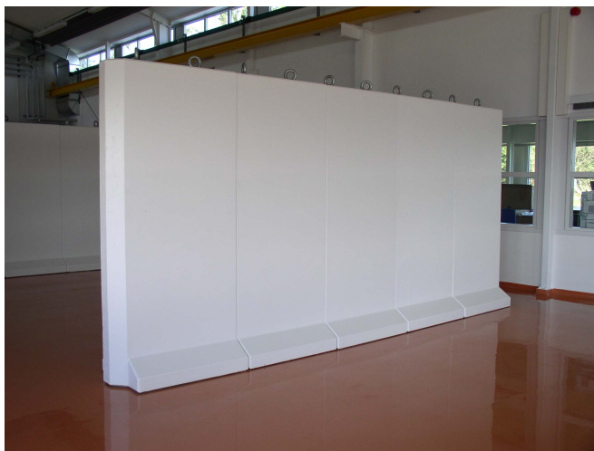
Figure 2. Measuring hall with shielding walls separating the germanium detectors. The shielding walls and the floor have been made of a special concrete with a very low content of ^{40}\text{K} , ^{238}\text{U} and ^{232}\text{Th} . The windows between the measuring hall and the control room can be seen in the background.
