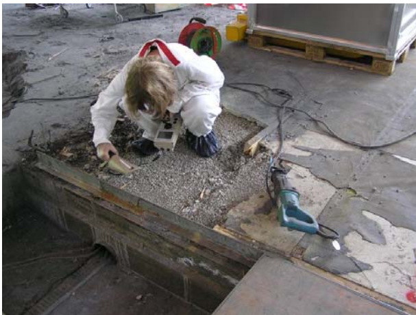
Figure 48 Checking for contamination in the sub floor.
