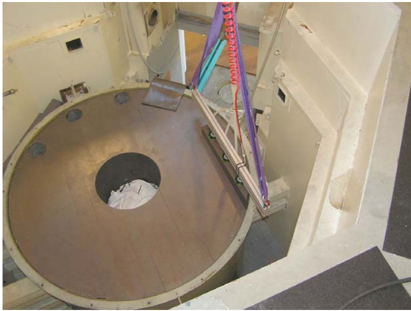
Figure 17 Beam with suction pads
