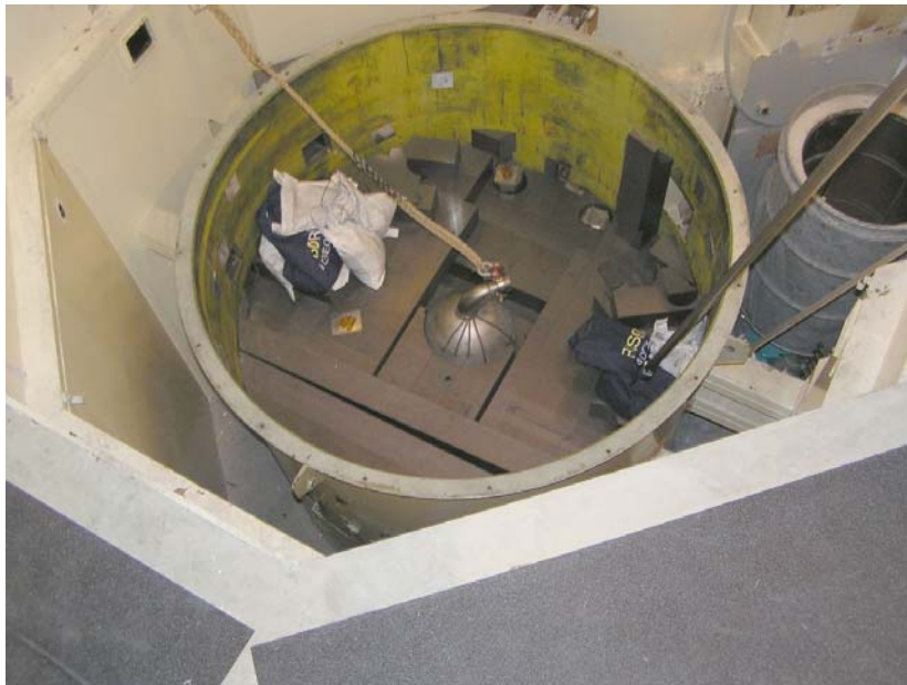
Figure 20 The core vessel ready to be lifted out
