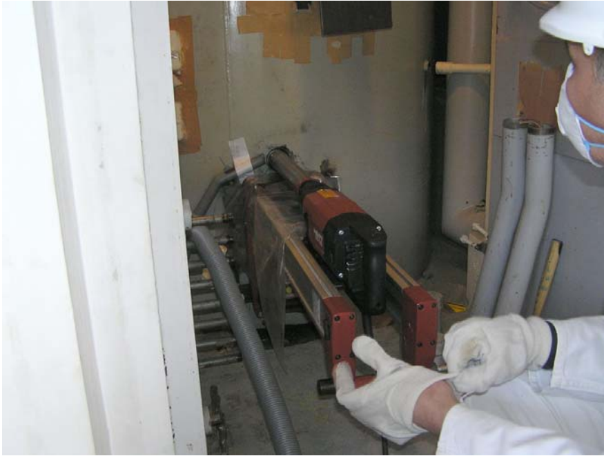
Figure 16 Drilling a core around the drainpipe
