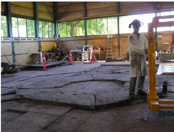
Figure 40 The foundation of the reactor block
