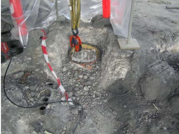
Figure 52 The collar on top of the FDT pipe being lifted out
