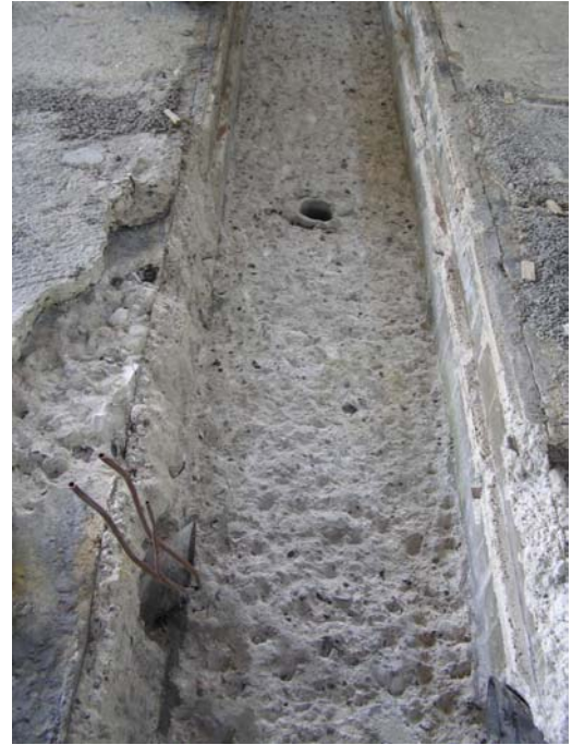
Figure 61 The southern channel after decontamination
