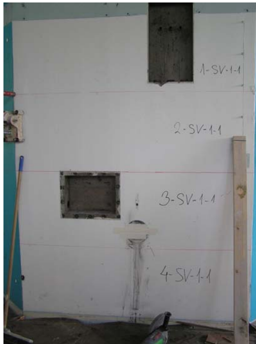
Figure 30 Horizontal cutting lines and block numbering on the south-western face
