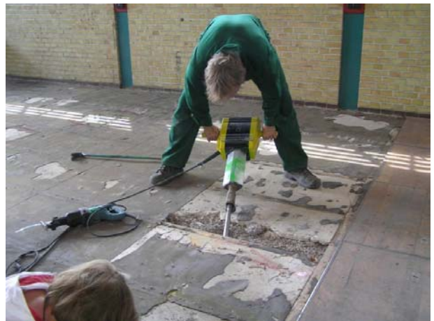
Figure 49 Removal of a contaminated area of the sub floor.
