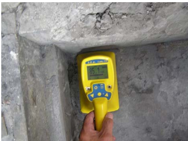
Figure 56 Contamination measurement in the northern channel, below the Fuel Mix Bowl
