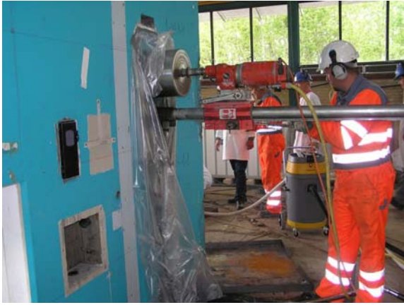
Figure 35 Channel on the western face being drilled out
