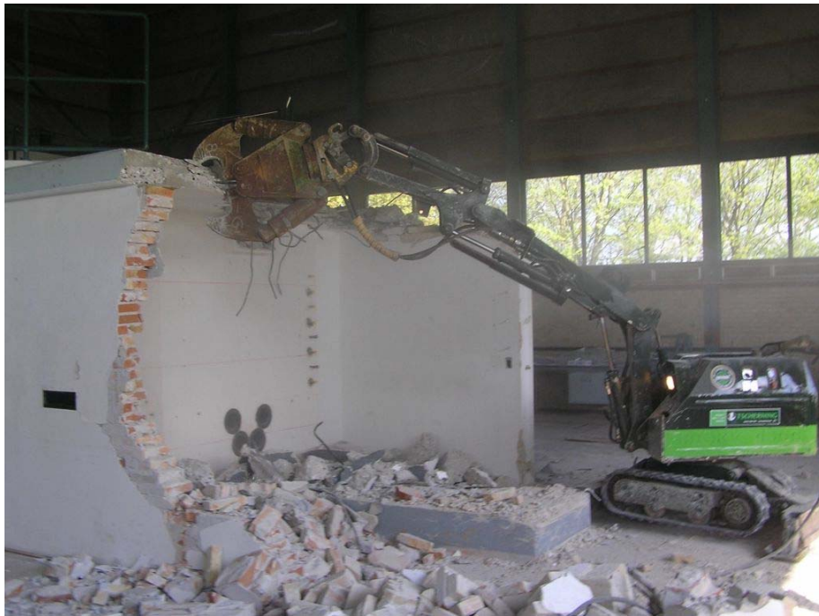
Figure 29 Demolition of the control rod house
