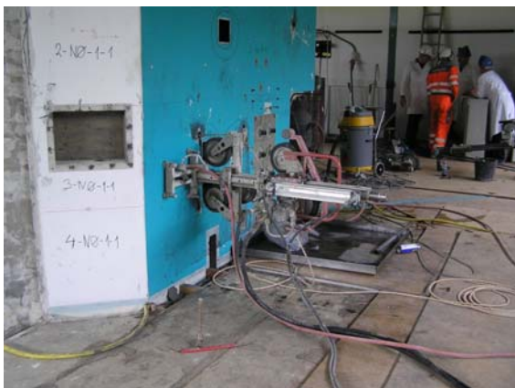
Figure 33 Cutting the four experimental channels on the northern face
