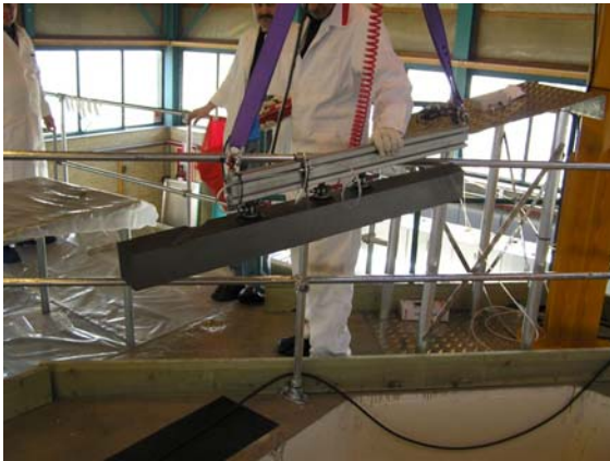
Figure 18 One of the longest stringers
