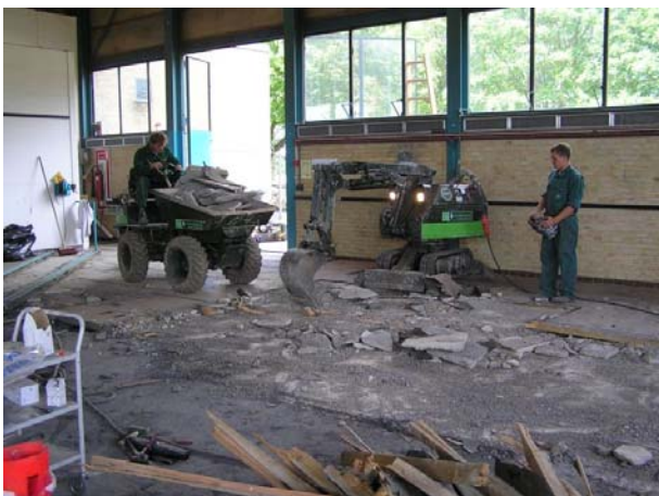
Figure 50 Removal of the sub floor
