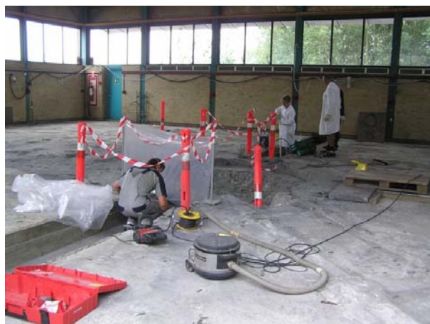
Figure 59 Decontamination work going on in the northern and the southern channel
