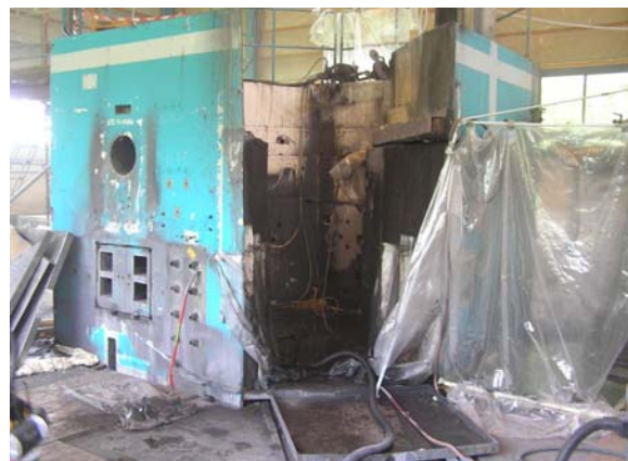
Figure 34 The block has been opened by cutting away the block above the "concrete door"
