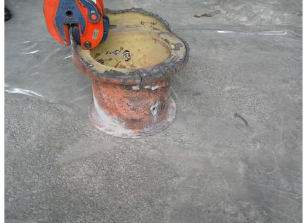
Figure 53 The collar with penetrations for ¼" pipes
