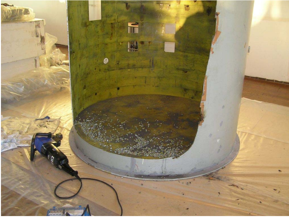
Figure 21 The nibbler and the half-cut reflector tank
