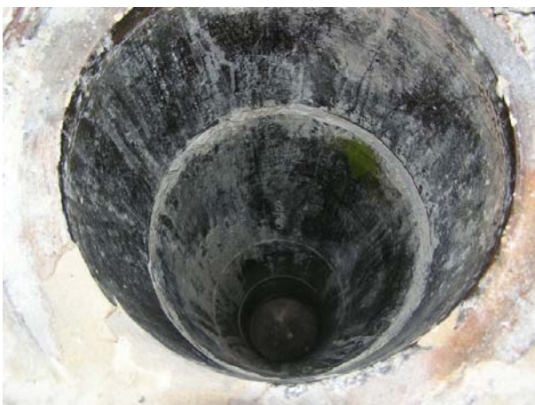
Figure 54 The pipe where the Fuel Drain Tank had been standing
