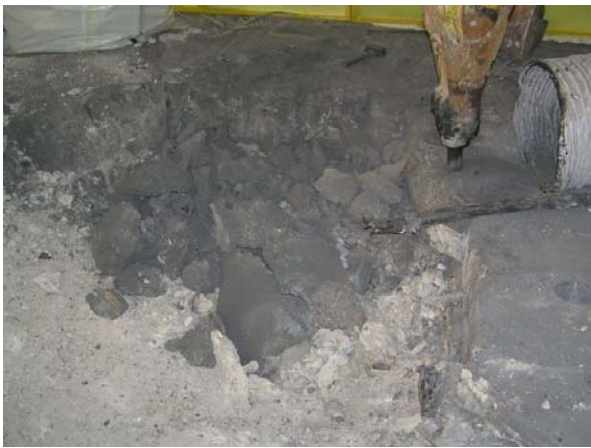
Figure 44 The central parts below the reactor being excavated
