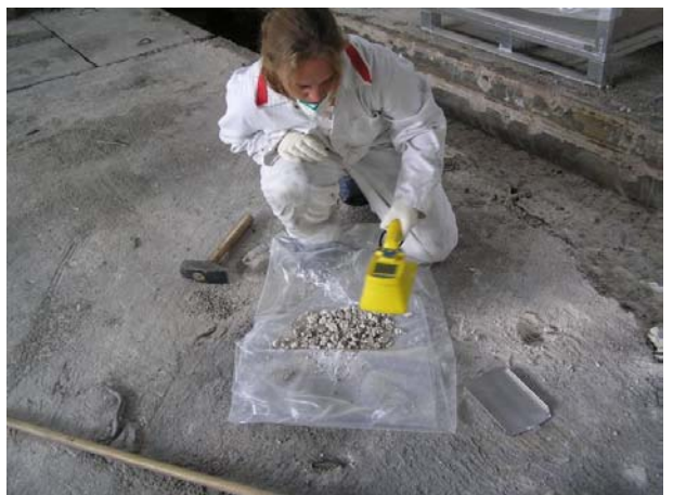
Figure 51 Checking that material from the concrete base is free of contamination.
