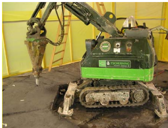
Figure 43 The Brokk demolition robot
