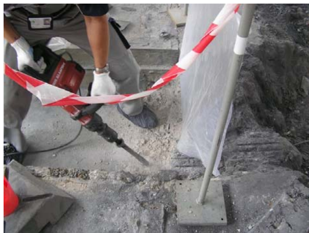
Figure 57 Contaminated concrete being chiselled away (northern channel)
