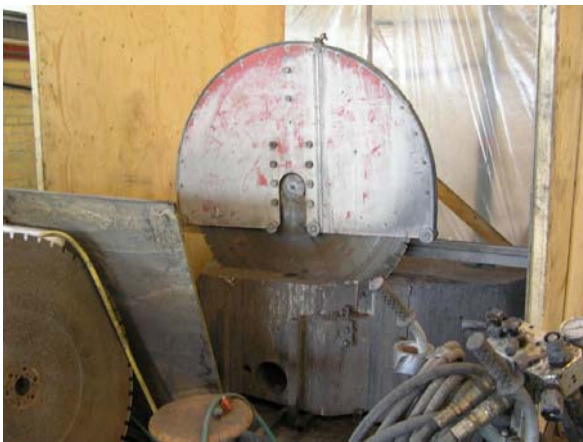
Figure 38 Circular saw cutting away the activated inner slab
