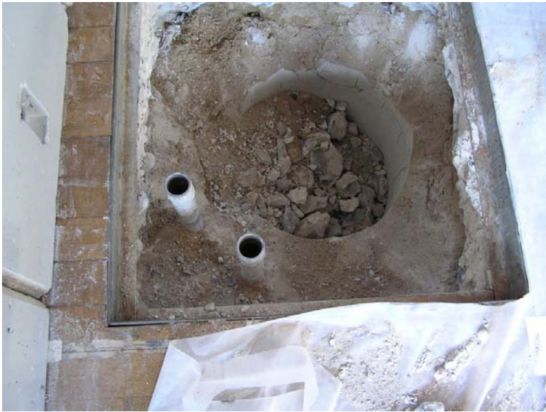
Figure 25 The well under the floor being demolished
