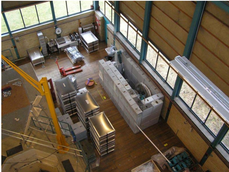
Figure 14 Photo taken from the overhead travelling crane. The shielded cell is seen in the centre of the photo.
