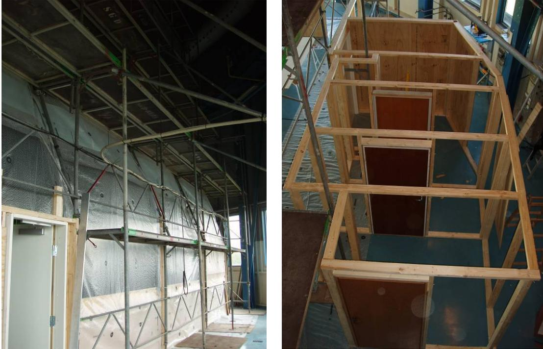
**Figure 45. Scaffolding covered with tarpaulin on the inside; three-section person lock being built.**
