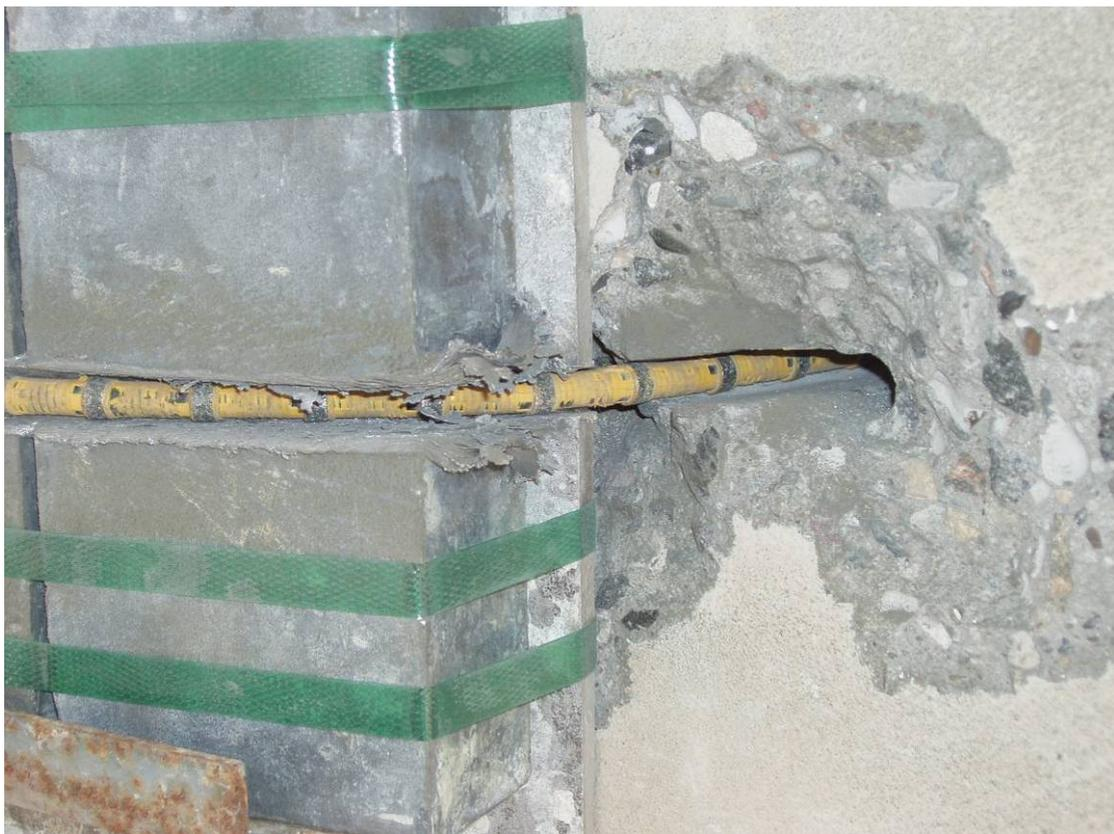
**Figure 58. Example of cutting lead using a wire.**
