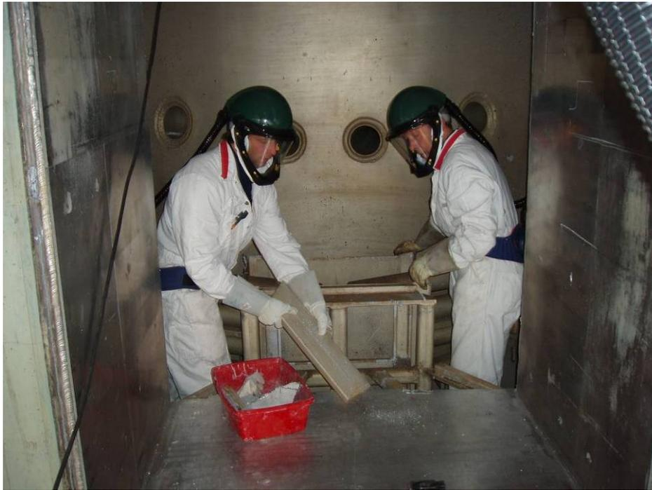
**Figure 36. The last internal parts of the reactor tank being removed.**
