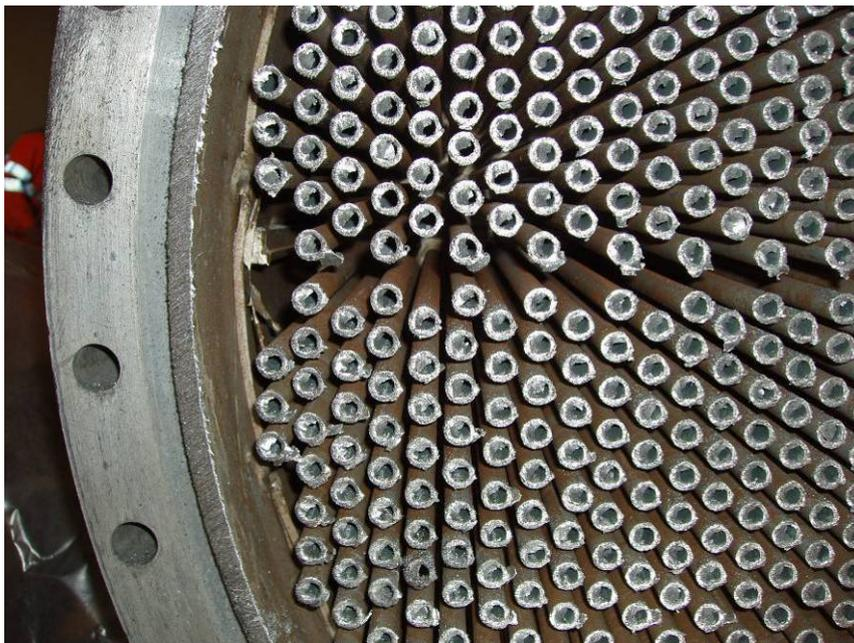
**Figure 40. Pipe ends in heat exchanger after dry wire-cutting.**
