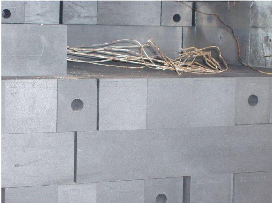
**Figure 25. Graphite stringers, cross bond visible, and cables for thermocouples in lead nose exposed.**
