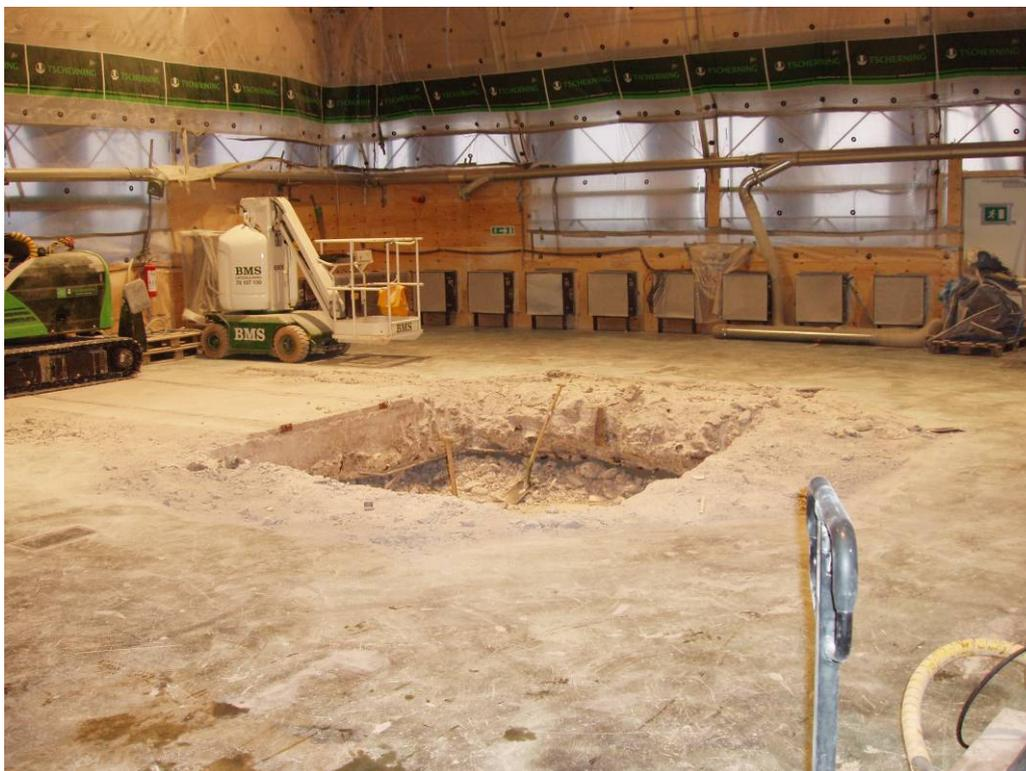
**Figure 67. The reactor has been removed. At the back is the southern tent wall with extraction units ("environmental boxes").**
