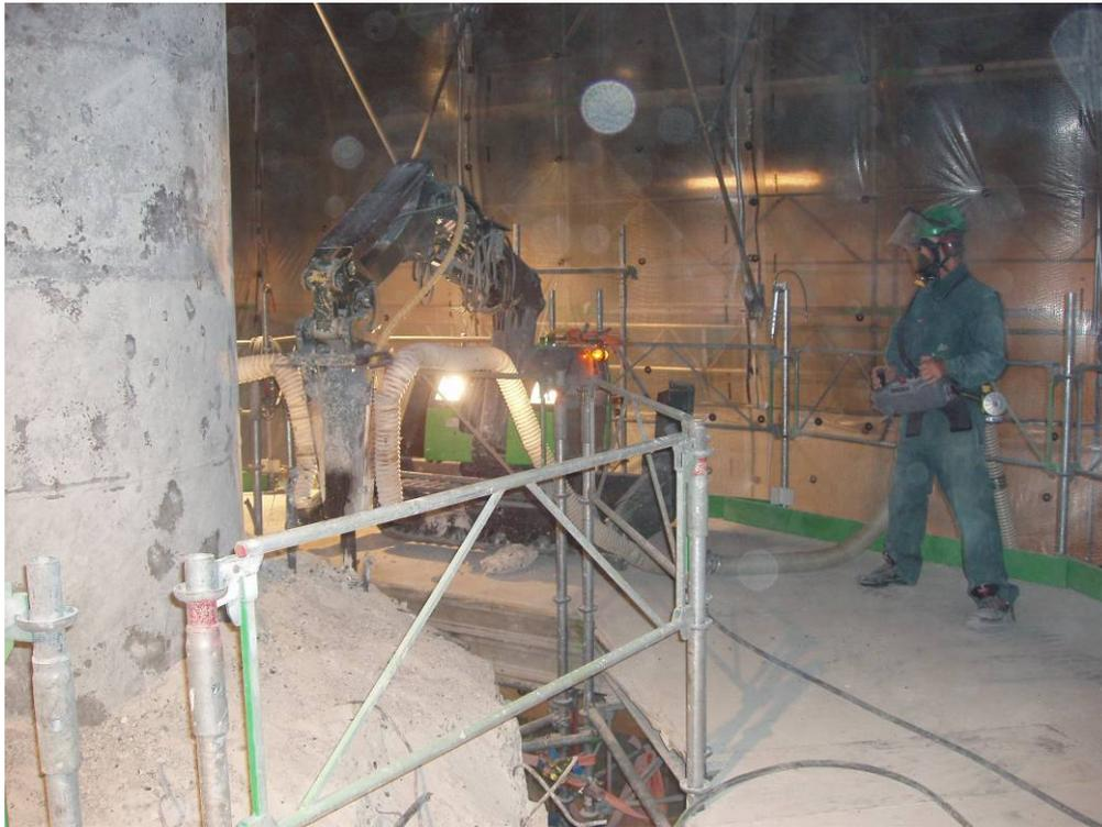
**Figure 52. Demolition of chimney from platform. Remote-controlled demolition robot 'Brokk90' in action.**
