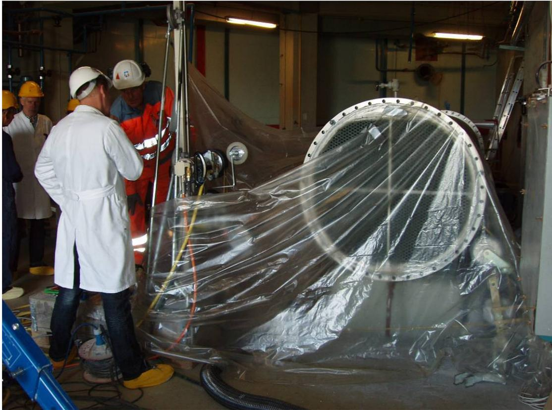
**Figure 39. Set-up for dry wire-cutting of heat-exchanger pipes.**
