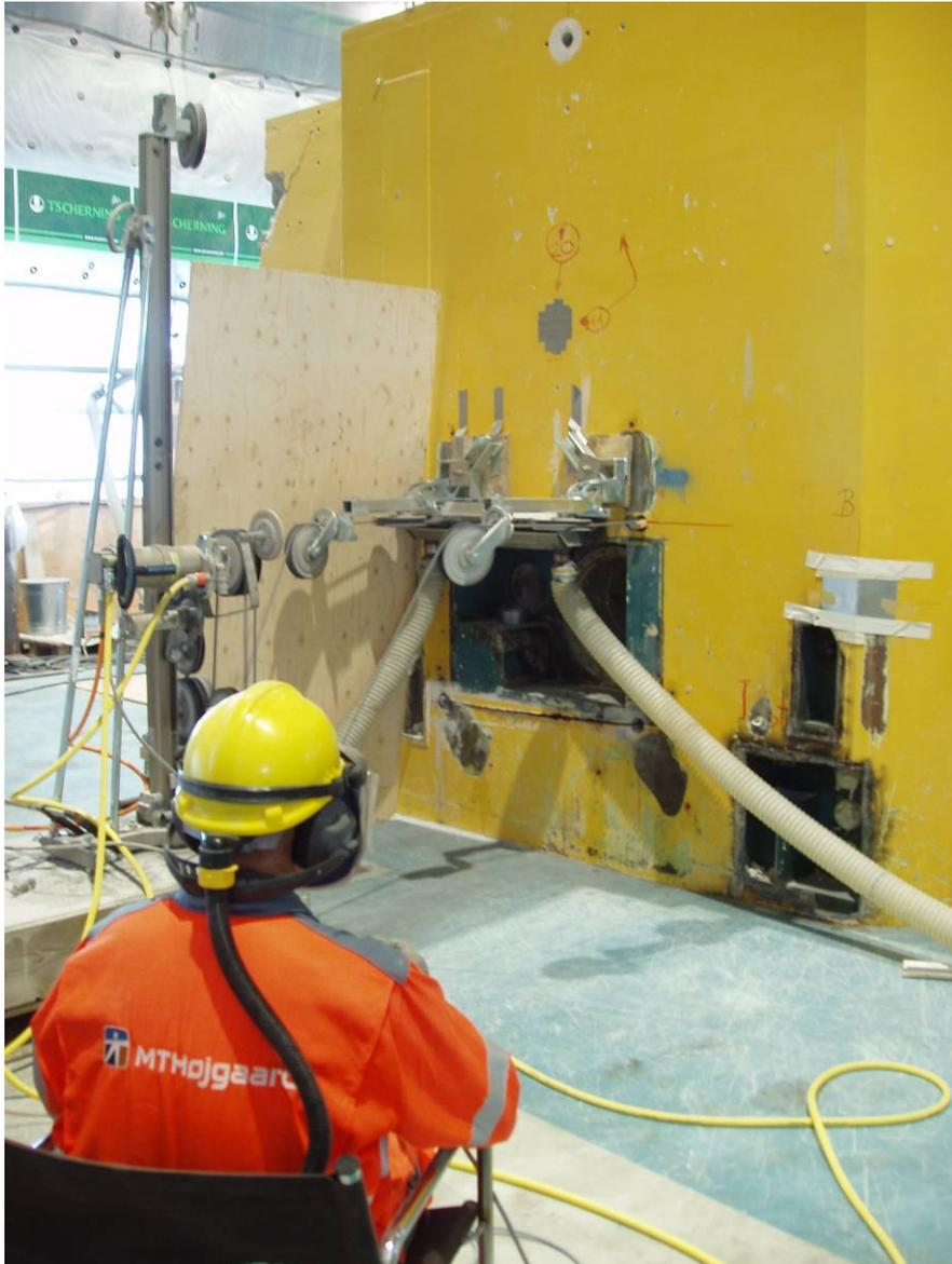
**Figure 59. Cutting of horizontal tubes using wire.**
