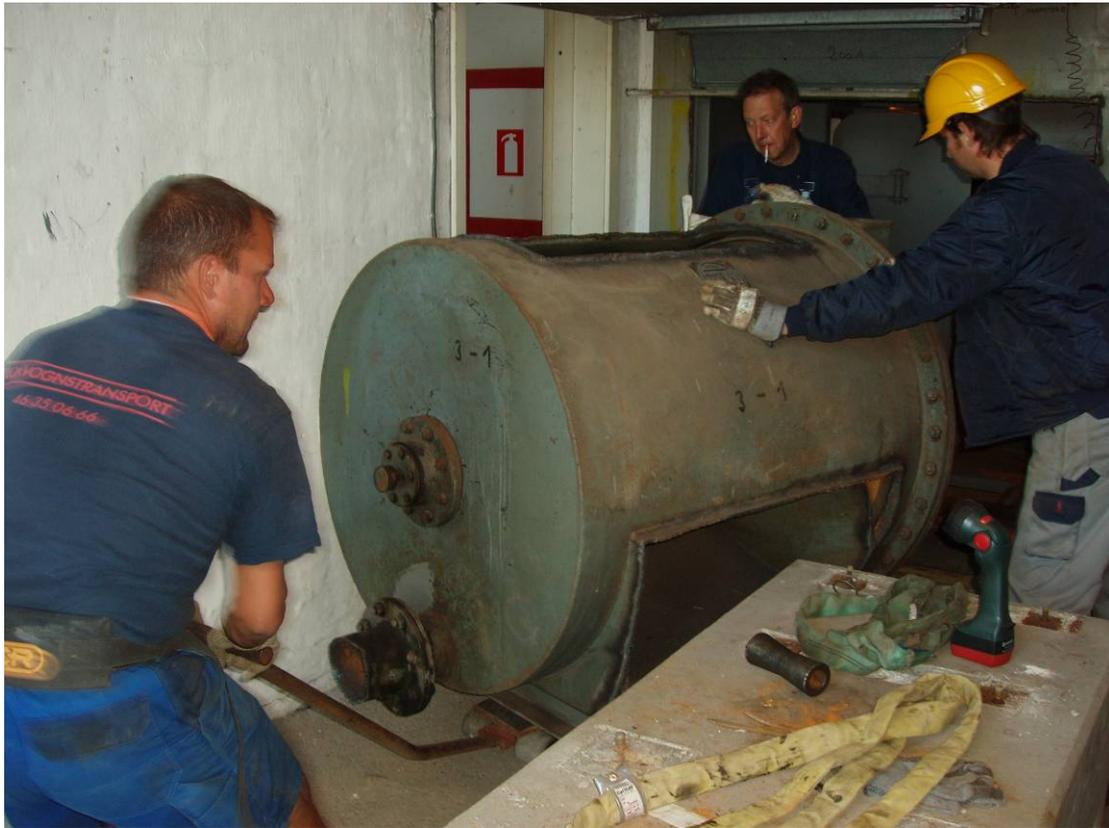
**Figure 9. Removing a Gako valve.**
