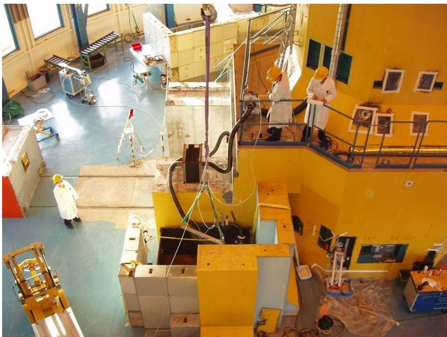
**Figure 26. Set-up for shielding and remote-controlled handling of graphite removal and container packing.**
