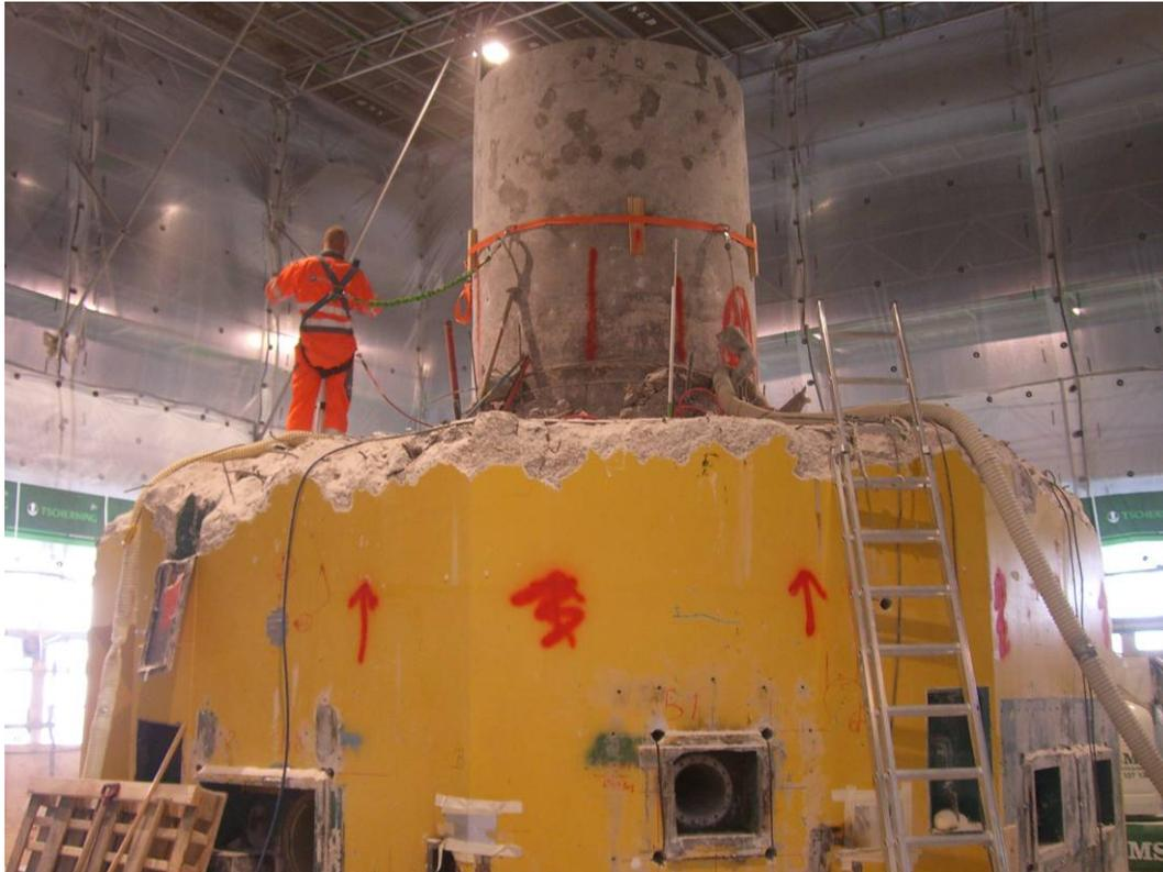
**Figure 56. Upper part of the reactor block broken up and preparations for cutting down the reactor tank.**
