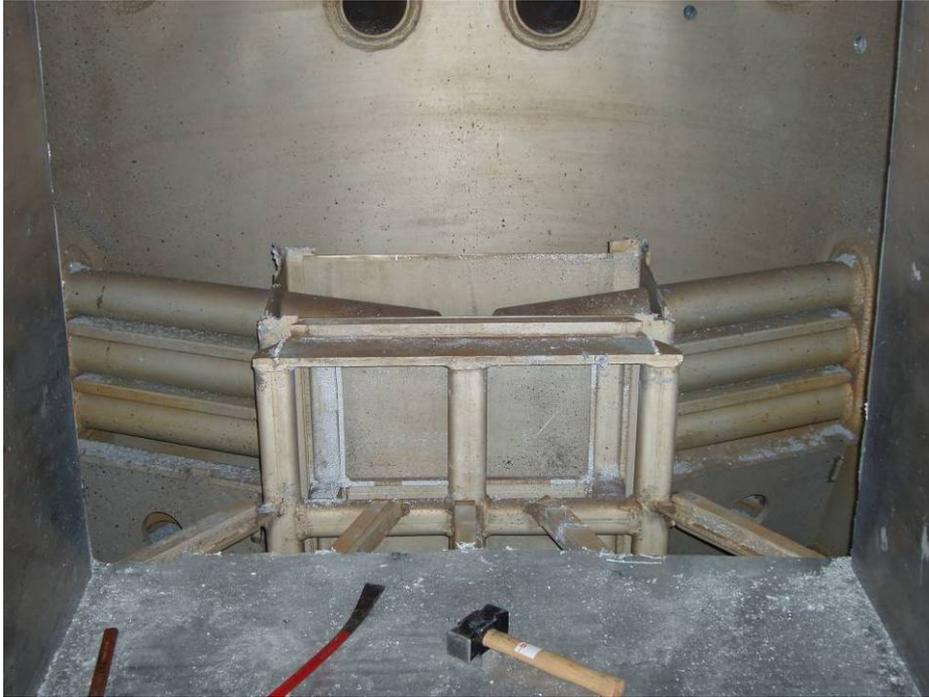
**Figure 35. The remaining inside structure after removal of the grid plate. Lead covers on instrument thimbles have been removed.**
