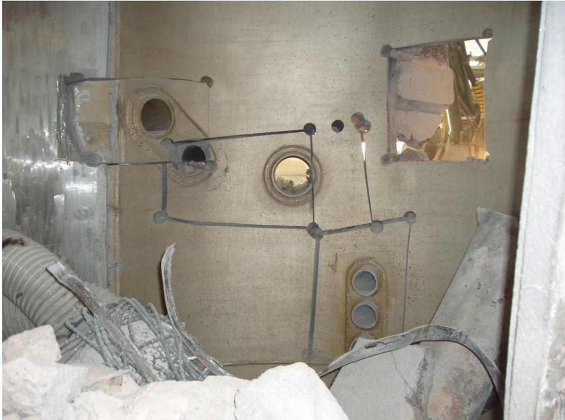
**Figure 61. Reactor tank seen from the inside during the cutting of horizontal tube blocks.**
