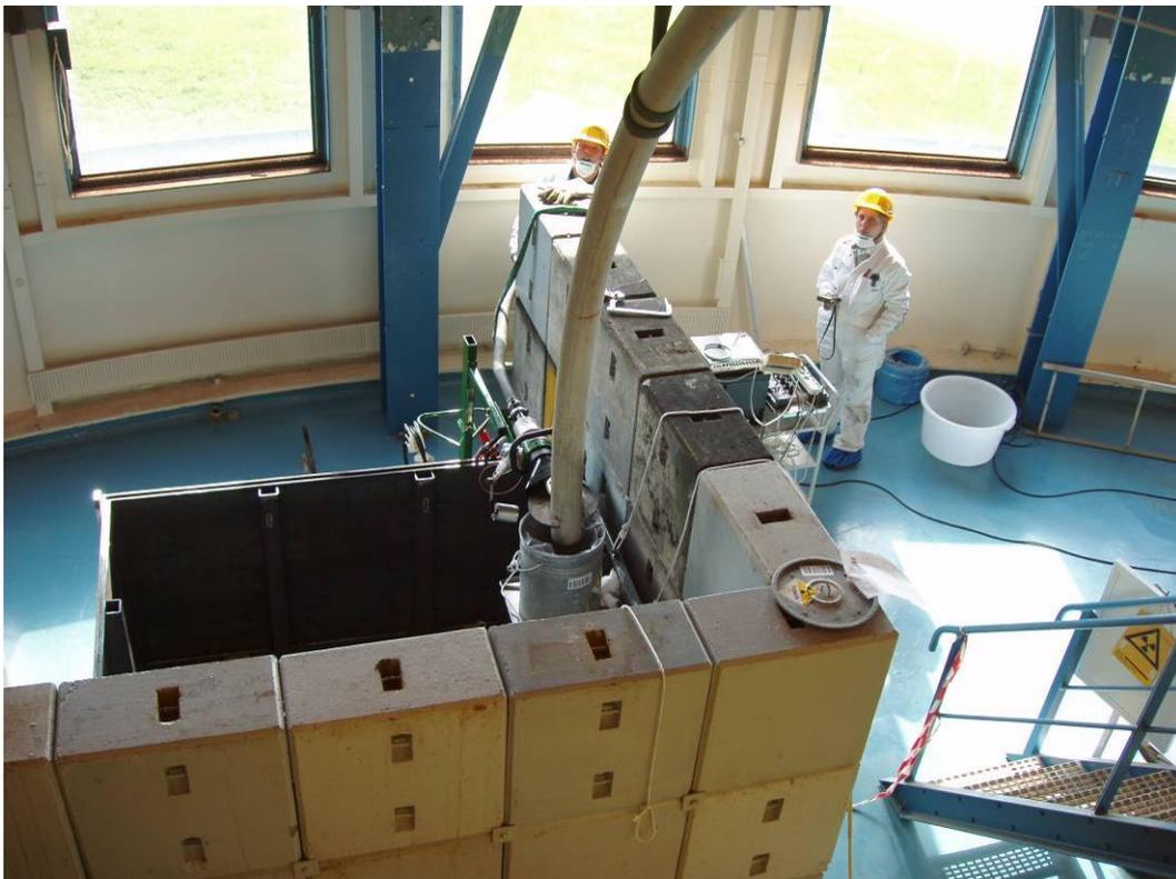
**Figure 22. Placement of remote-controlled shear above container. A camera has been mounted on the shears themselves. The monitor is outside the shielding.**
