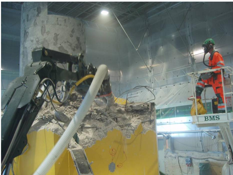
**Figure 55. Demolition of upper part. Demolition robot 'Brokk330' remote-controlled from the lift.**
