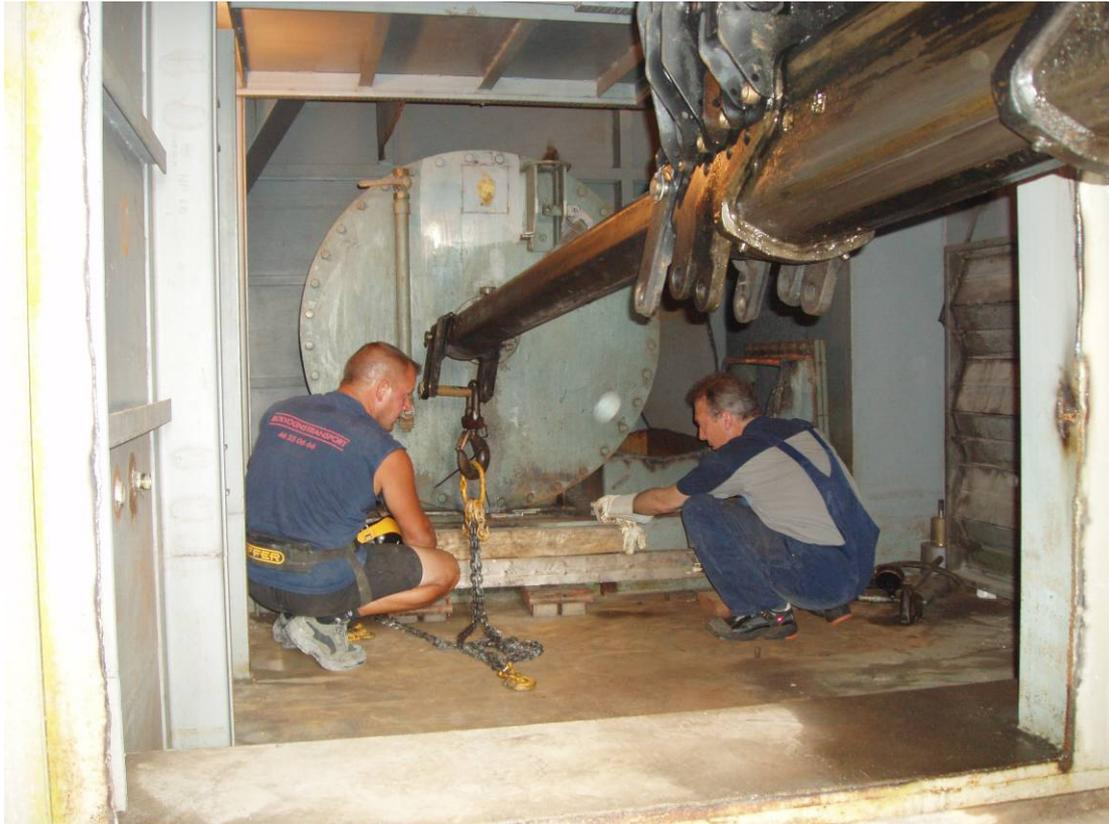
**Figure 8. Preparing to remove a Gako valve.**
