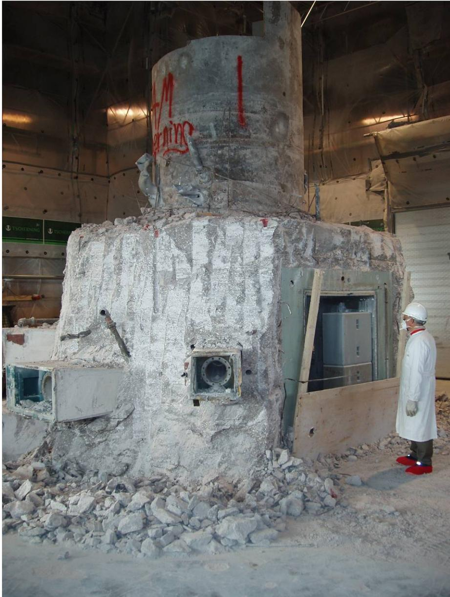
**Figure 63. Process step 5 completed. Activated concrete part “exposed”.**
