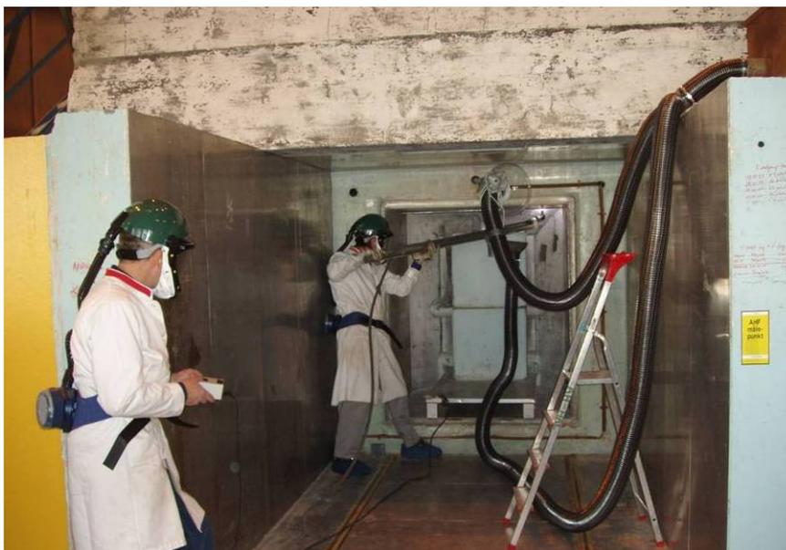
**Figure 30. Plasma cutting of lead nose. Shielding with concrete blocks at the centre; local air extraction used.**
