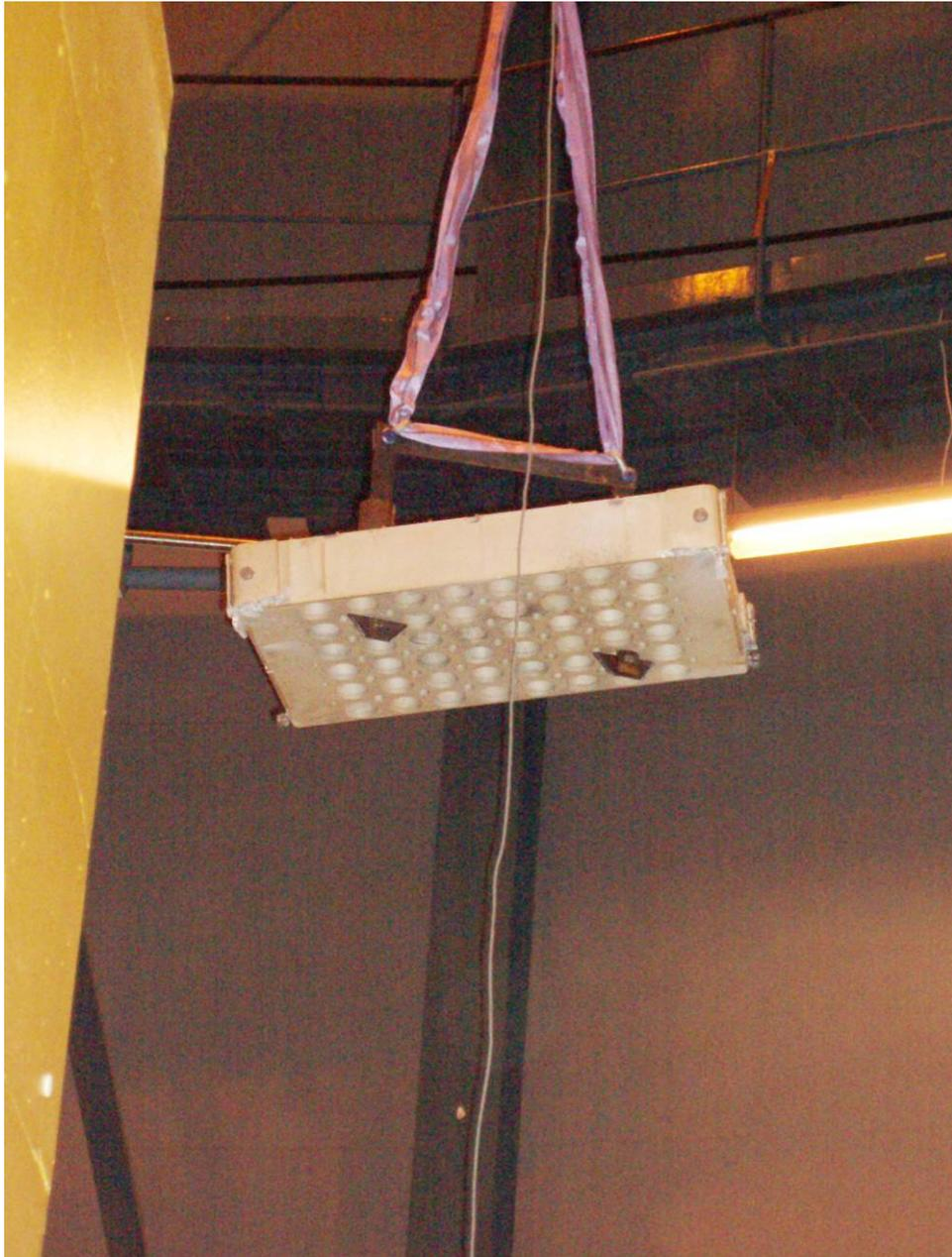
**Figure 33. The grid plate being lifted out of the reactor tank. The lifting bracket and steel bolts at the corners are visible.**
