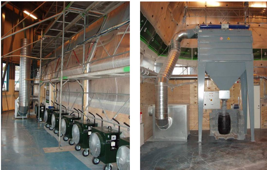
**Figure 46. Left photo: extraction system on the discharge side; at the back discharge from a local extraction point. Right photo: system for local extraction with a drum for collecting dust; discharge via HEPA filter.**
