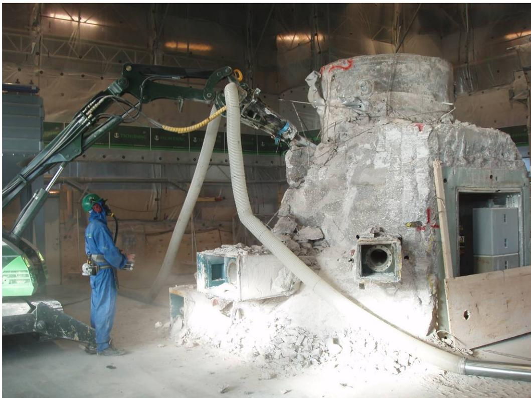
**Figure 65. Demolition of activated part of reactor block. Local extraction system fitted on a hydraulic hammer.**
