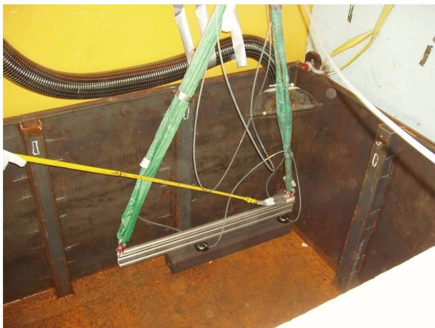
**Figure 27. A graphite stringer being removed by using a vacuum lifting device and placed in a DD steel container.**
