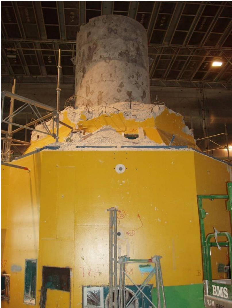
**Figure 53. Chimney broken up; platform is removed; reactor tank awaits cutting up.**
