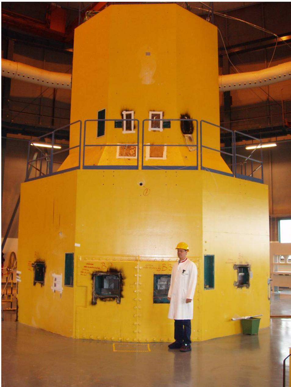
**Figure 6. Reactor block and project manager at the commencement of the decommissioning process (June 2006). Access apertures for experiment tubes are concealed.**
