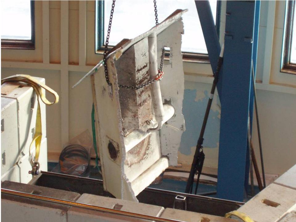
**Figure 31. Lead nose cut off and placed in a container.**
